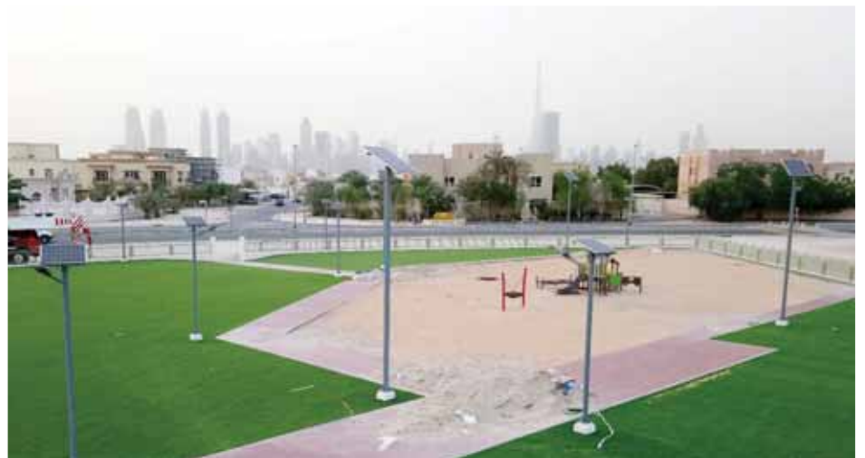
END USER: DUBAI MUNICIPALITY LOCATION: AL-QUOZ, DUBAI SYSTEM: 50W SOLAR STREET LIGHT
